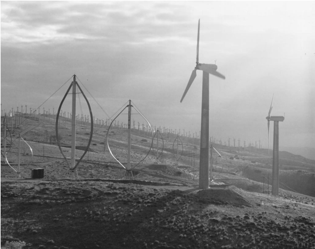
FIGURE 8.11.2 Wind farm both horizontal-axis and vertical-axis turbines.
